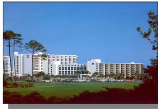
Sandestin Hilton Expansion / Addition — Sandestin, FL
